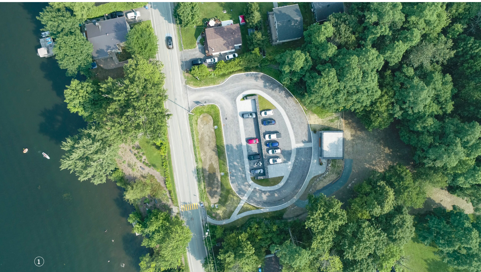
1. The Carke Terrace seen from the air. The installations have been built on a large lot on both sides of Bondville Road, offering a third public access to Brome Lake.
